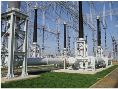
An electrical substation in China is using high temperature superconductor (HTS) wire. Located in the city of Baiyin in the Gansu province of China, and built by the <a href="Institute of Electrical">Institute of Electrical</a>
